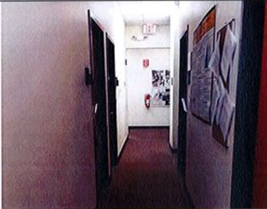
21. Corridor width not 48" ADA compliant.
