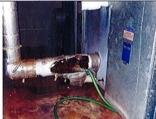
24. More corroded piping in HVAC mezzanine.
