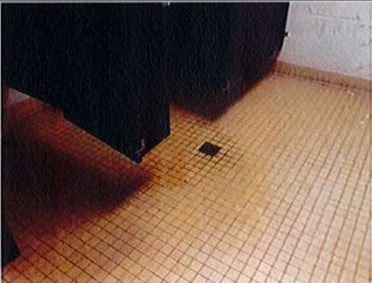
17. Drains clogged in unused restroom.
