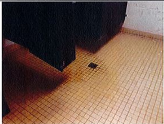
17. Drains clogged in unused restroom.
