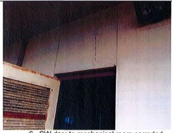
6. SW door to mechanical room corroded and crack over door.
