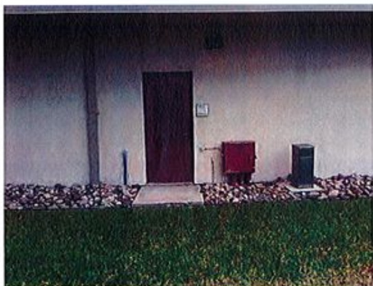
5. SW door to mechanical room.
