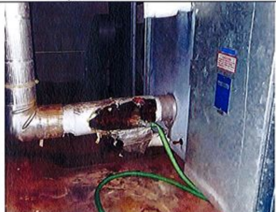
24. More corroded piping in HVAC mezzanine.
