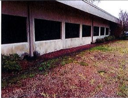
1. NE exterior side showing extensive mildew buildup from moisture.
