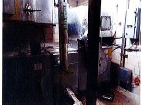
14. HVAC unit in mezzanine.
