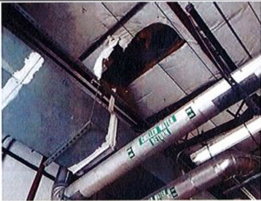
9. Roof area inside mechanical room.
