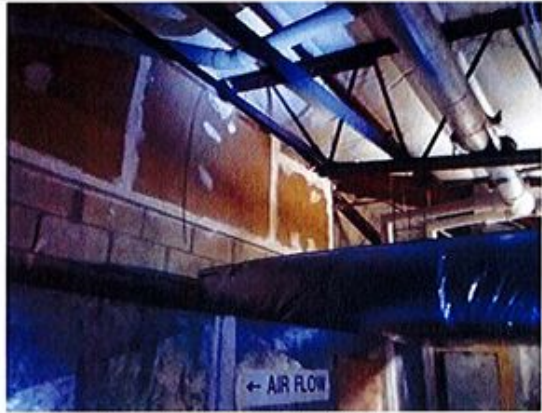
13. Roof in mechanical mezzanine.
