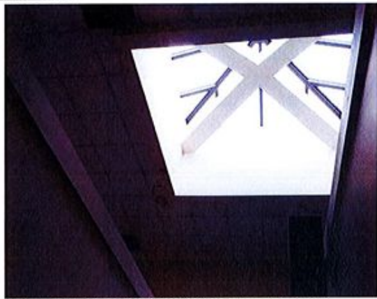
19. Apparent leaks in roofing around skylight.
