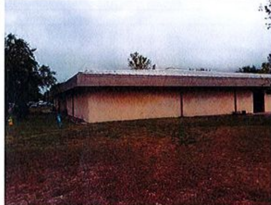
8. SE Corner of building.
