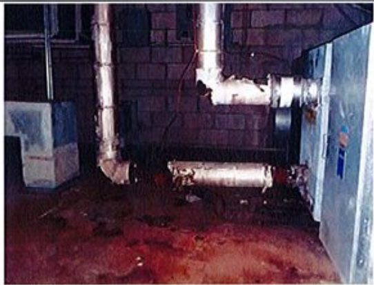
15. Corroded piping in mezzanine HVAC.
