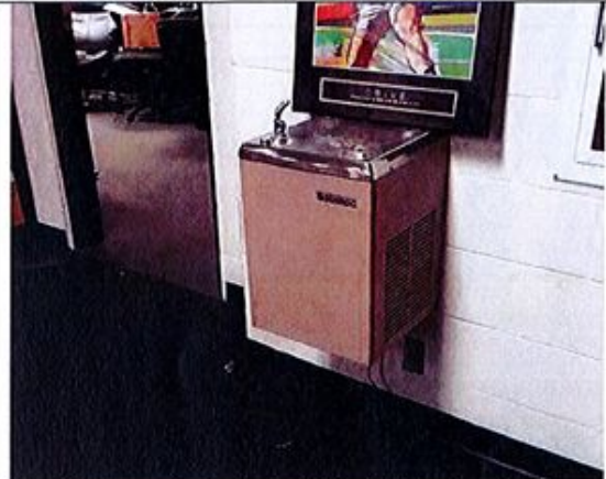
20. Non-compliant single ADA drinking fountain.
