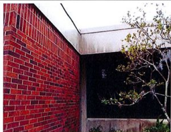
2. NE corner with mildew.
