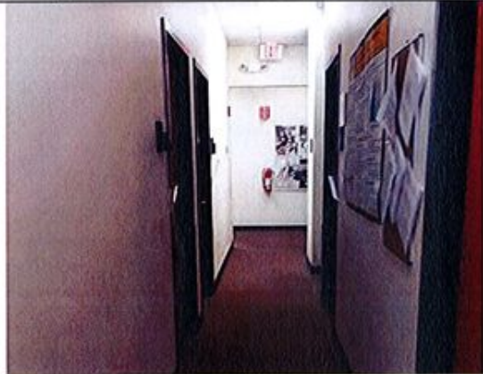
21. Corridor width not 48" ADA compliant.
