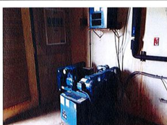
12. Mechanical room with moisture in walls.
