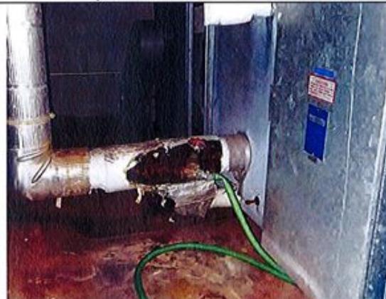
24. More corroded piping in HVAC mezzanine.
