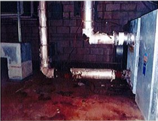
15. Corroded piping in mezzanine HVAC.
