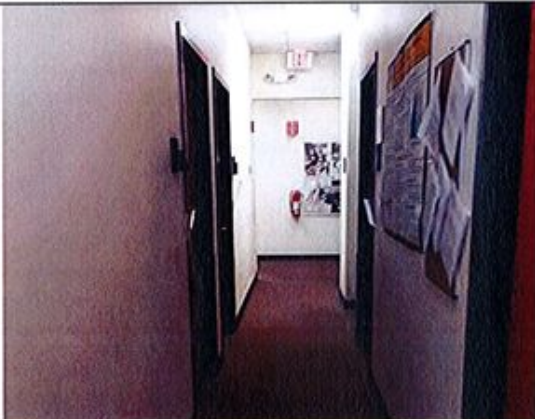
21. Corridor width not 48" ADA compliant.
