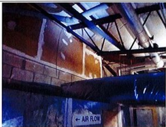
13. Roof in mechanical mezzanine.
