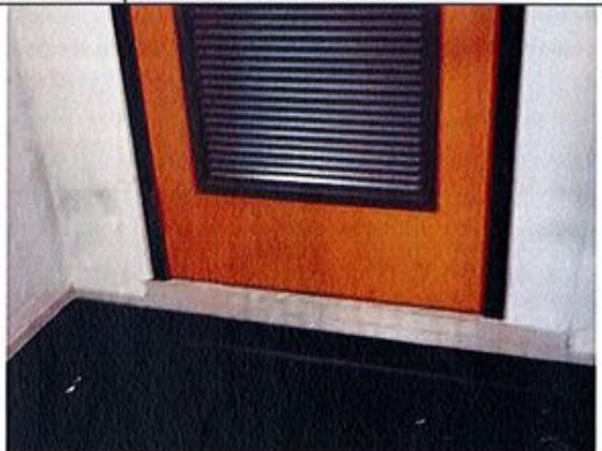
18. Step into shower room.
