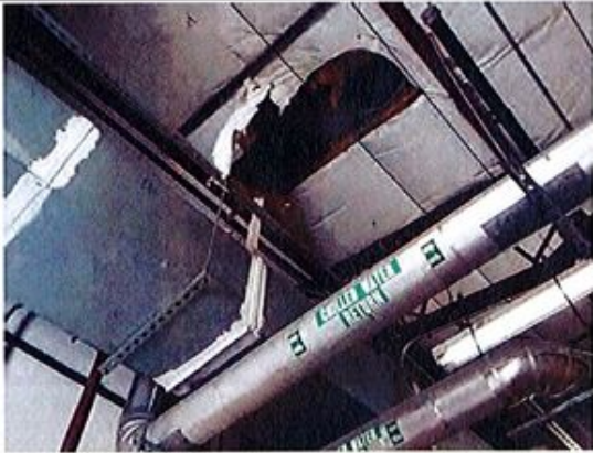
9. Roof area inside mechanical room.
