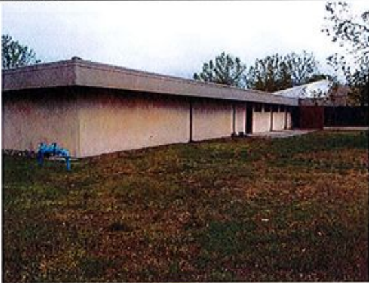
7. SE side of building.
