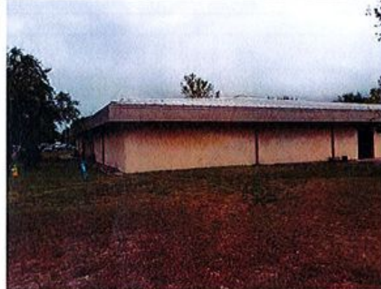
8. SE Corner of building.
