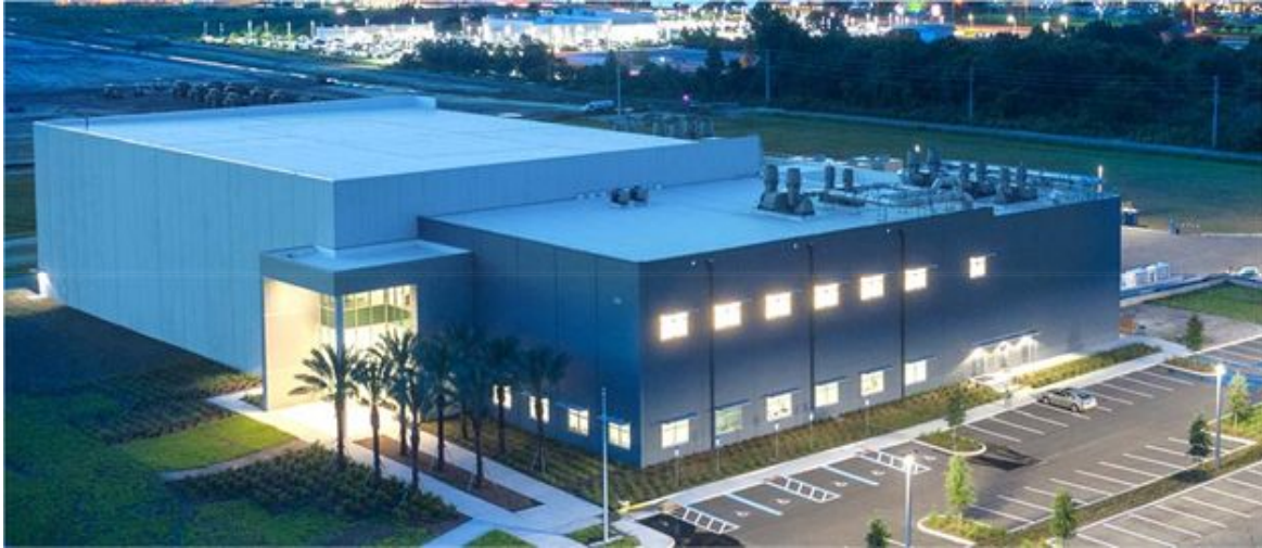
BRIDG Facility – August 2017
