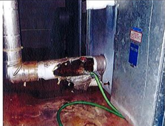
24. More corroded piping in HVAC mezzanine.
