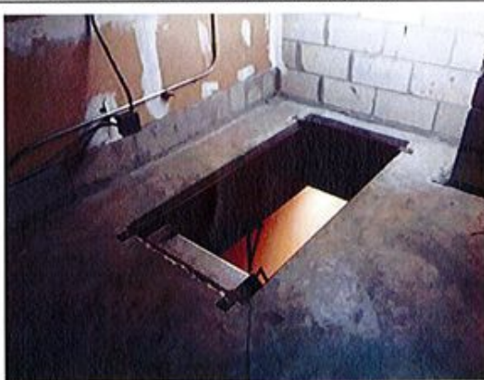
23. No railing around access to mezzanine.
