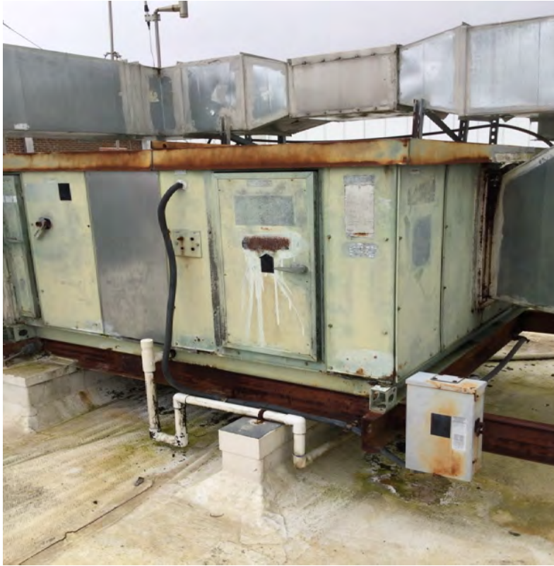
CREOL Research B0053 - roof AHU 5-6 (1989 Original) – FCA 2025 Time Frame A. Est. cost of $700k
