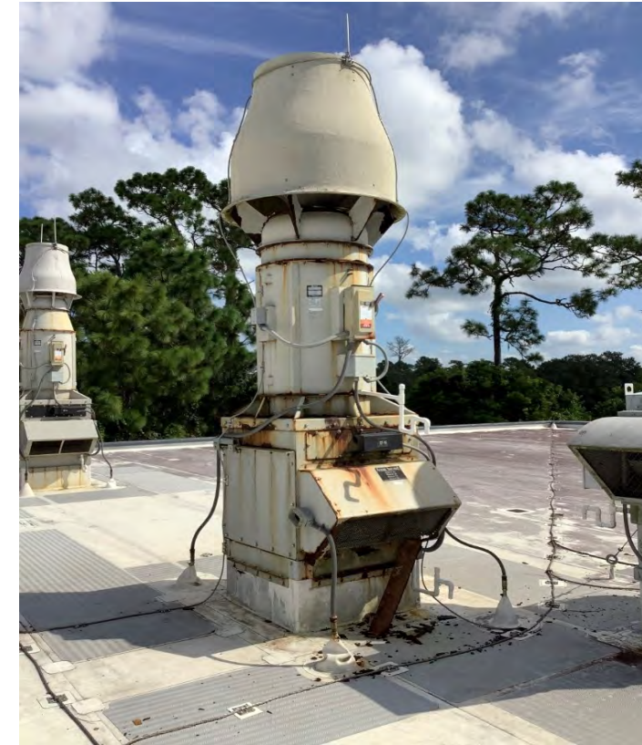
Mechanical, Materials and Aerospace Engineering B0154 – Roof laboratory exhaust systems replacement – FCA Deferred Maintenance. Est. cost $300k
