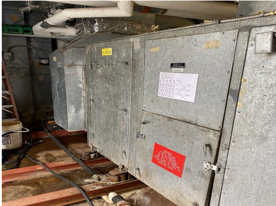
Theater B0006 - AHU-2 (1982 Original to building) – FCA 2025 Time frame A. Est. cost $816k
