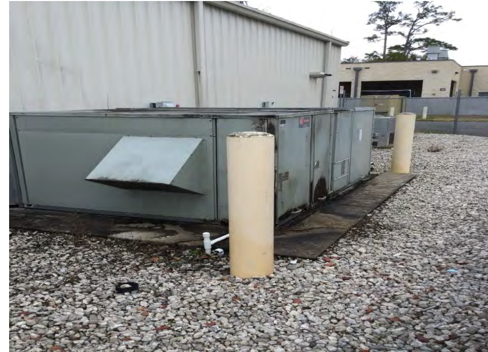
Siemens Research B0044 - PU DX-2 (2010 Original to building) – FCA 2025 Time frame A. Est. cost $115k
